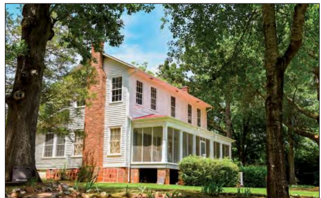
Plantation house at Andalusia Farm near Milledgeville, Georgia, where O'Connor lived and wrote for much of her life. It is now on the National Register of Historic Places. Georgia College & State University
