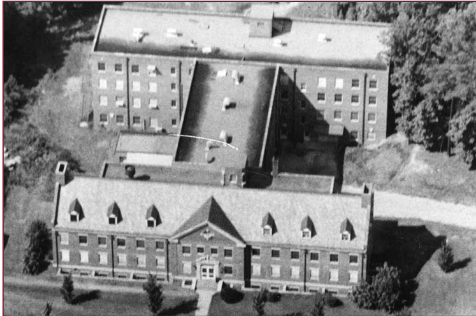
The Bell Building.
